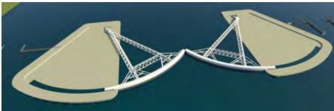
Figure 1: Floating Sector Gate and Artificial Island
