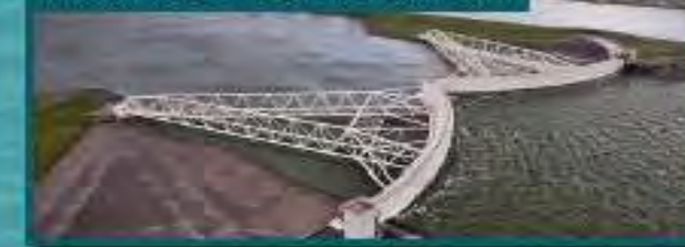
Maeslant Storm Barrier Rotterdam
